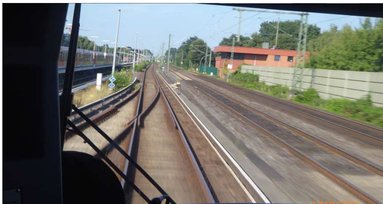
transition 3rd rail to catenary
