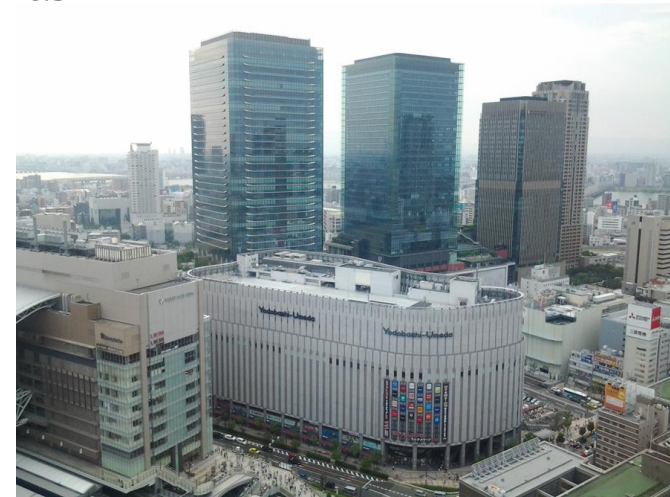
Grand Front Osaka buildings
