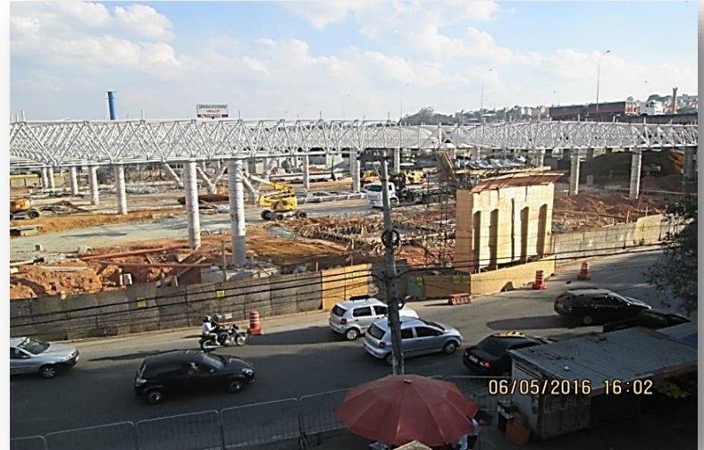
Terminal Osasco km 21
