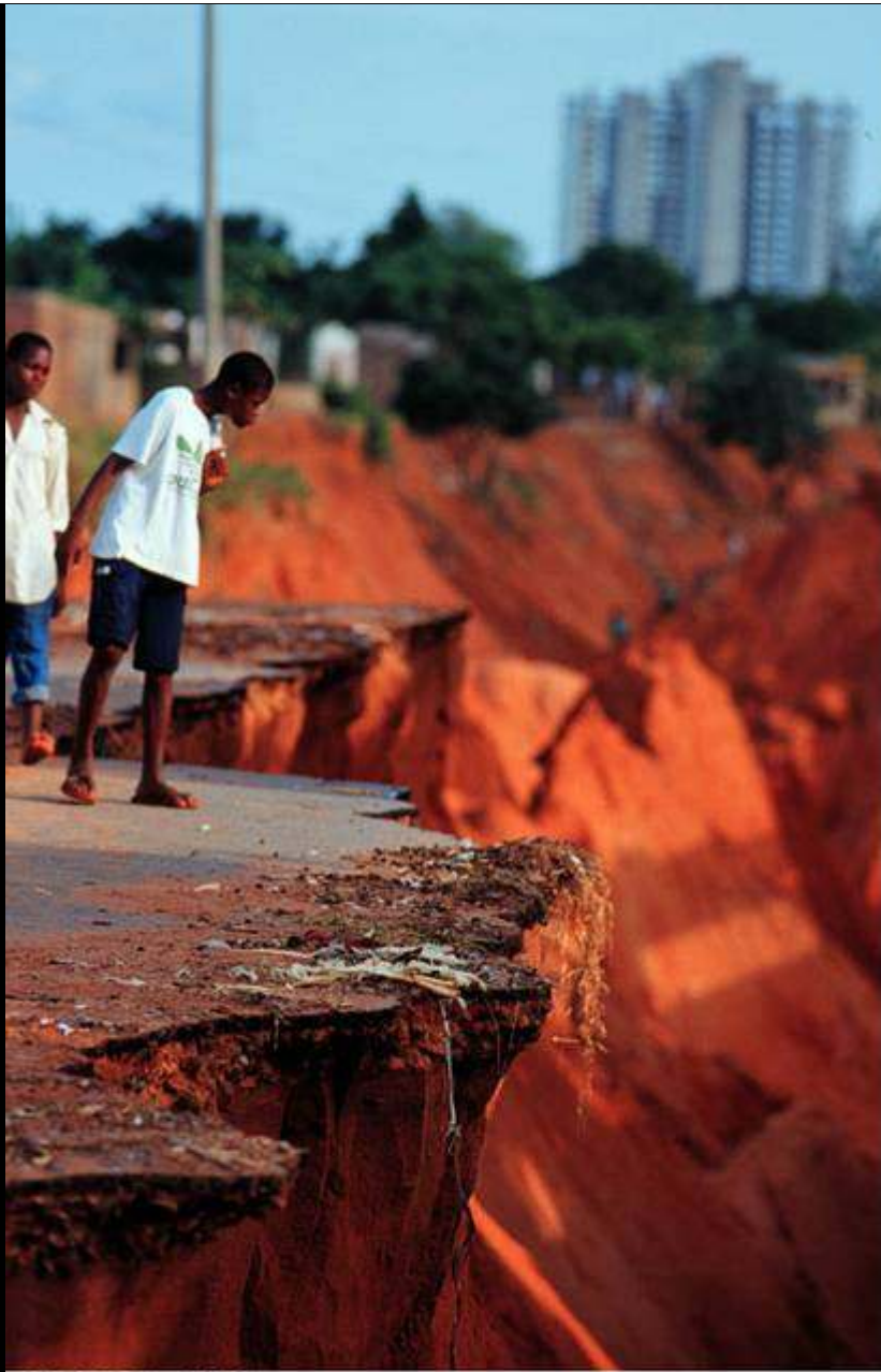
17 MARCH 2003 Torrential rains slice a massive gorge into the capital city. The road and 100 homes were lost, Mozambique Accession. ©Greenpeace/Shirley
