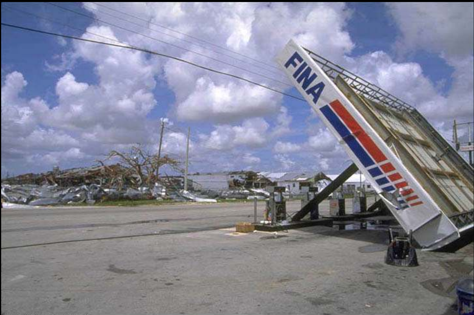
1 AUGUST 1992 Damage caused by Hurricane Andrew, Dade County, Miami, Florida. USA. ©Greenpeace/Perrine
