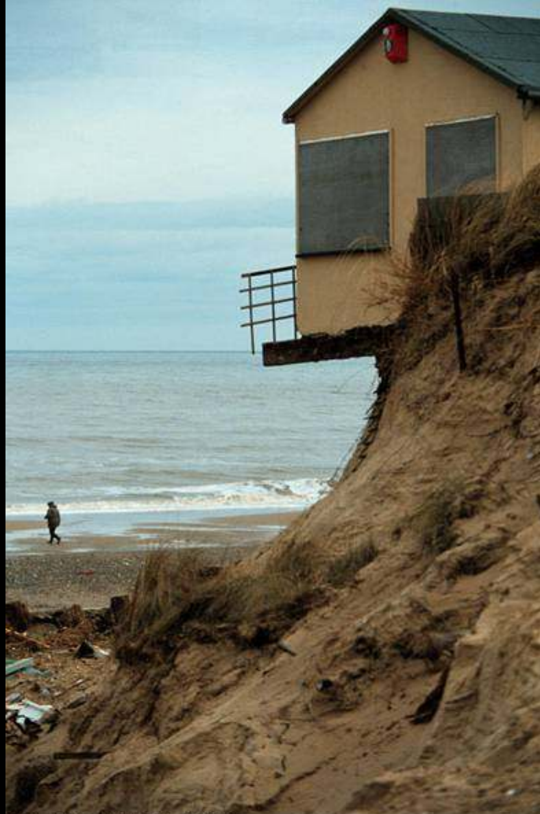
23 FEBRUARY 1993 Holiday chalet in danger of collapse as high tides and wave pressure erode the sand, Hemsby, Norfolk. East coast England. ©Greenpeace/Hodson
