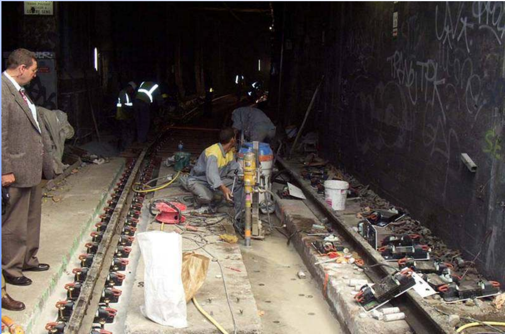
Valhubert tunnel - Paris
