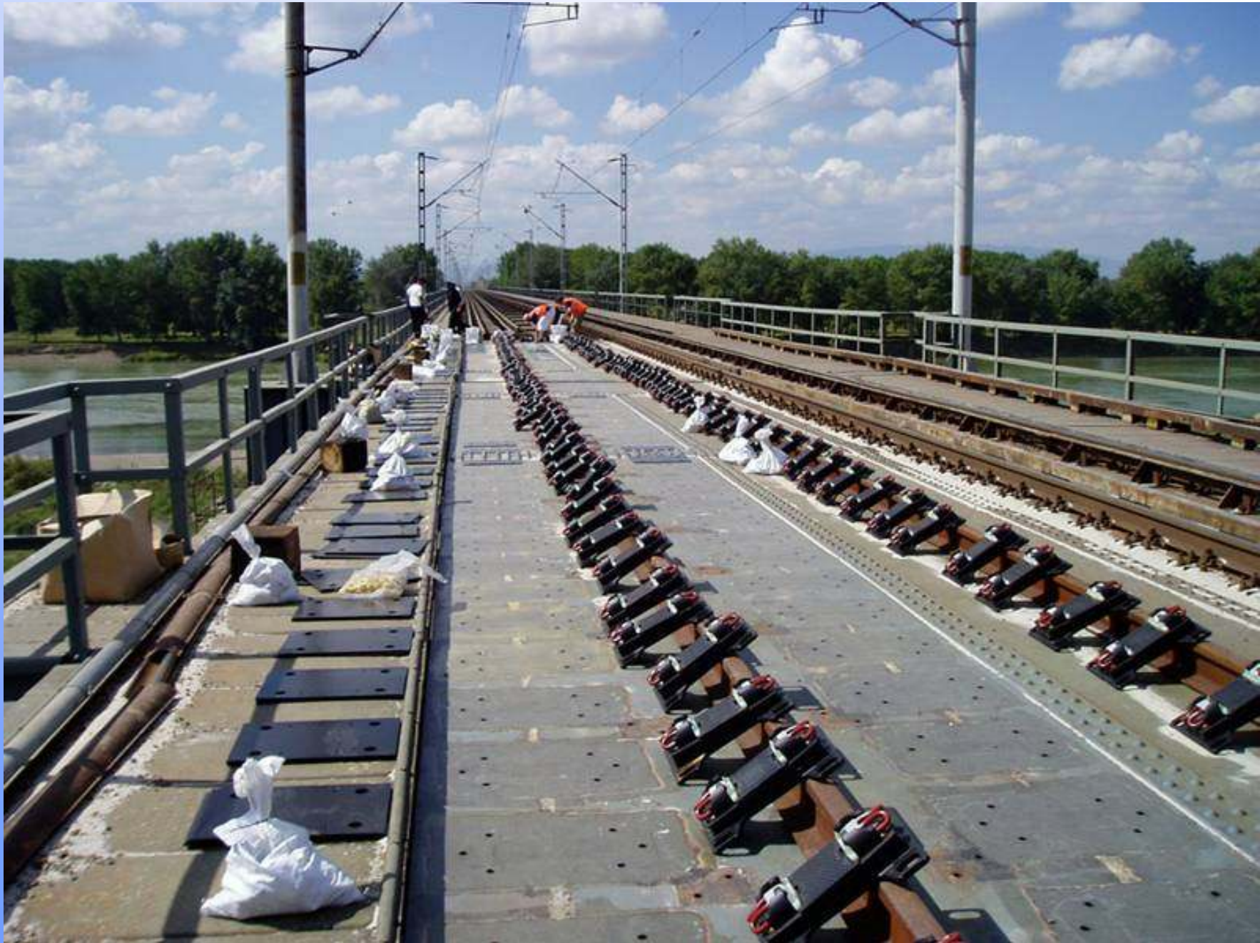
Cosmesti Bridge - Romania
