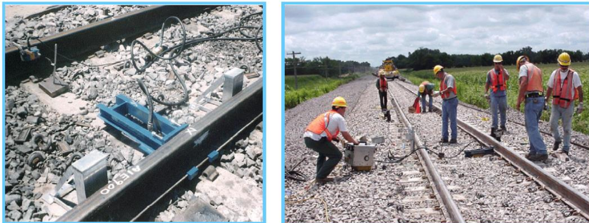
Single Tie Push Test (STPT) Measurement
