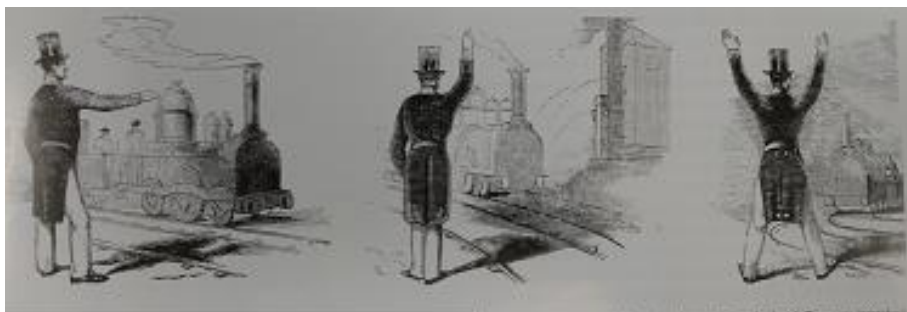
Above: In the absence of flags, signals were given by hand. One arm stretched out horizontally meant 'line clear', one arm raised meant 'caution', both arms raised meant 'danger stop'. These same clear and danger hand signals were also used in France, Spain and the USA. In Britain the clear and caution hand signals exchanged meanings in the mid-1920s. Illustrated London News
